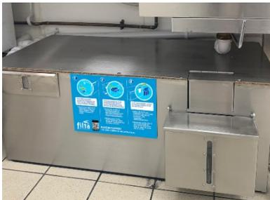
Image 3: FiltaFOG Cyclone grease recovery unit
